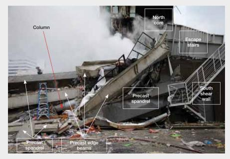
Figure 59(b): Spandrel panels and edge beams to the west of the south shear wall (source: Robert Heywood)
