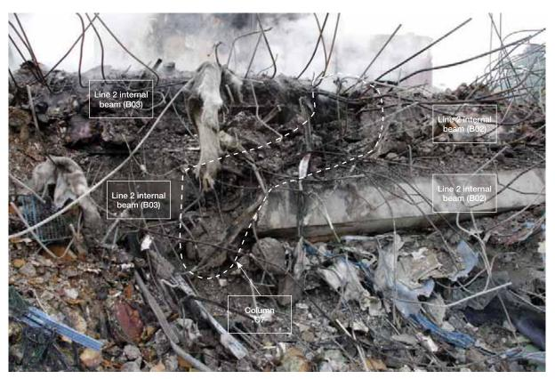
Figure 62(h): The junction between line 2 and column C7 looking north towards the north wall complex. The remains of column C7 are in the centre (source: Robert Heywood)
