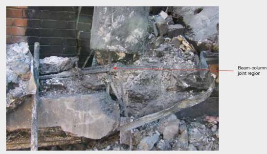
Figure 64(a): Disintegrated beam-column joint (source: Graham Frost)
