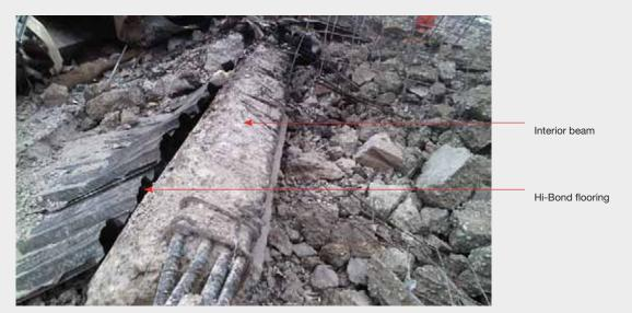
Figure 63(b): Interior beam from the western side of the building (source: Graham Frost)
