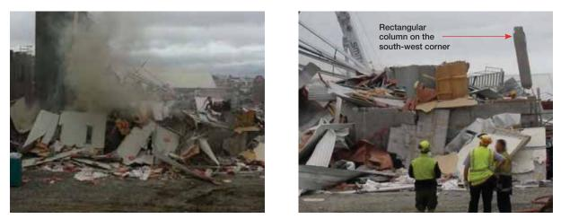
Figures 62(d) and (e): The western elevation with the column on the south-west corner visible (source: Hyland/Smith<sup>1</sup> report)
