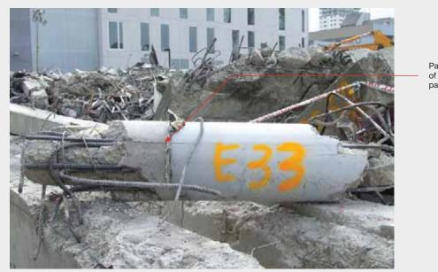
Paint line at the top of where the spandrel panel abutted
