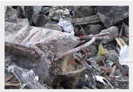
Section from which the corner or "wing" has broken away
