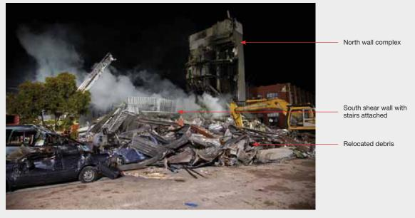
(b) North wall complex and collapsed south shear wall with relocated material in the foreground at 4am on 24 February 2011 (source: Robert Heywood)
