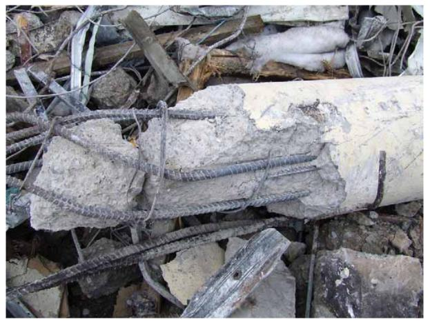
Figure 62(c): Column of unknown location showing vertical reinforcing bars and spiral transverse reinforcement. Concrete has spalled off from outside the reinforcement and fractured inside (source: Graham Frost)
